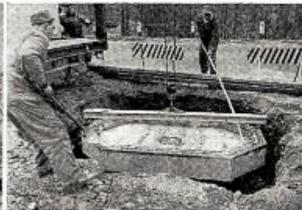
Lower manhole vault . . .
